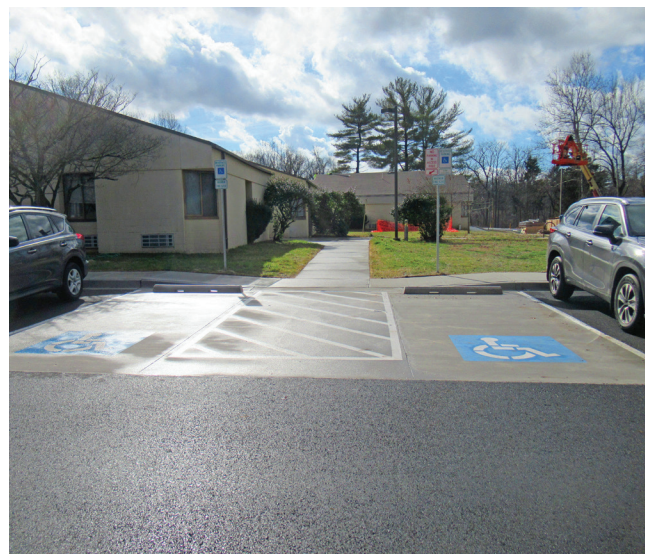
Avery Rd. ADA Parking
