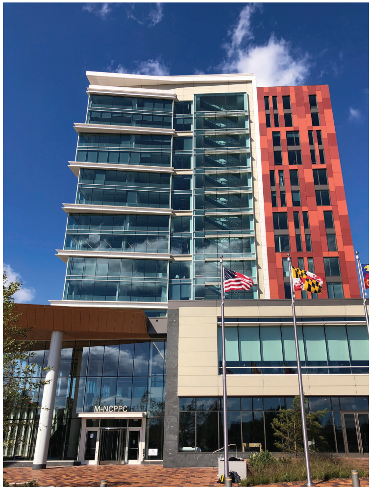
Wheaton Office Building
