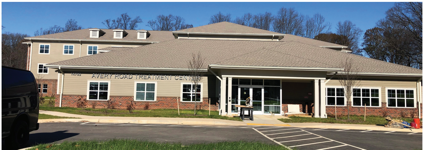
14703 Avery Road Treatment Center
