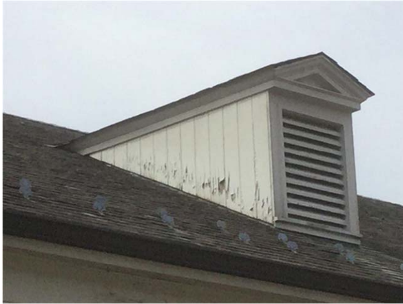
Photo 9: Dormer shown in Photo 8. Note the peeling paint.
