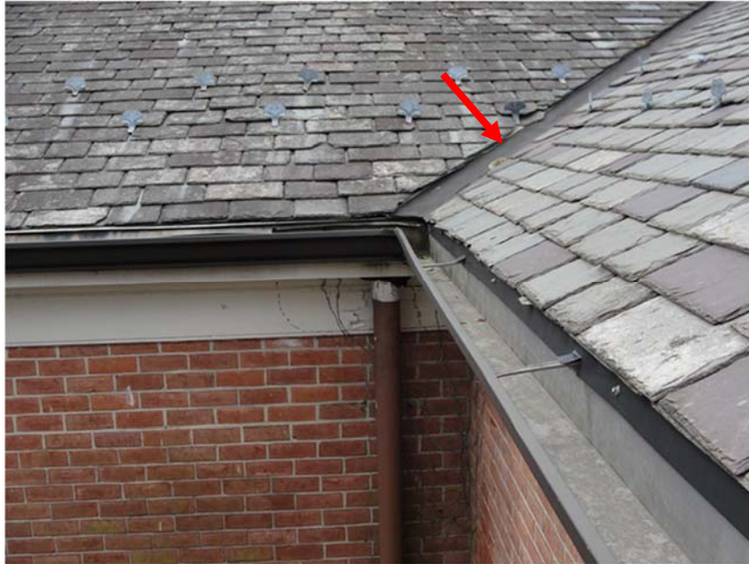
Photo 7: Typical sheet metal hung gutter assembly. Note EPDM membrane repairs observed in valley (red arrow).
