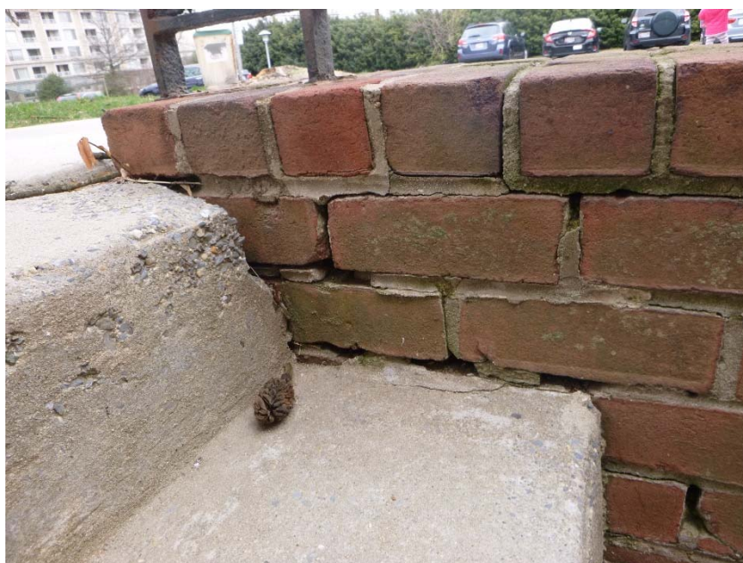
Photo 12: Deteriorated mortar on the north retaining wall.
