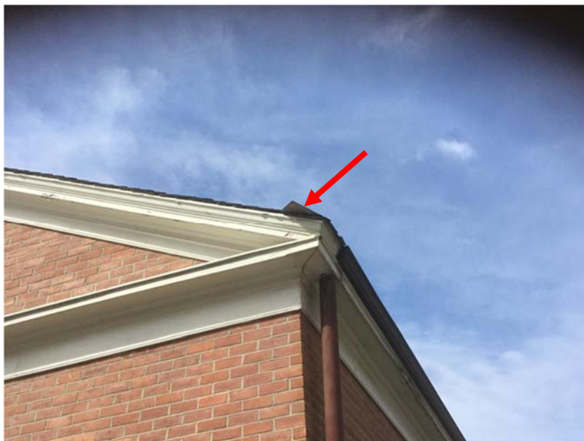
Photo 6: Slate shingle displacement along the roof edge (red arrow).
