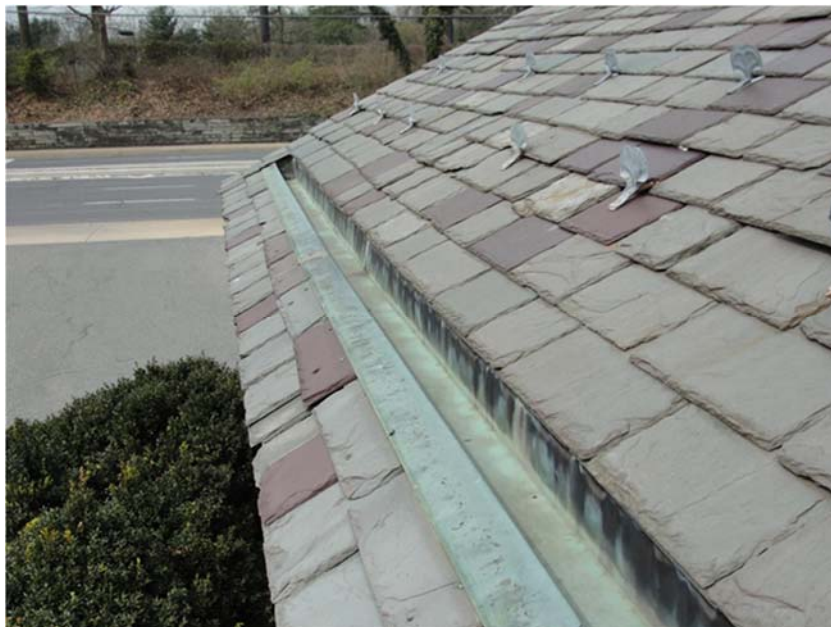
Photo 4: Typical copper built-in gutter assembly. Isolated damaged slate tiles noted at this edge.
