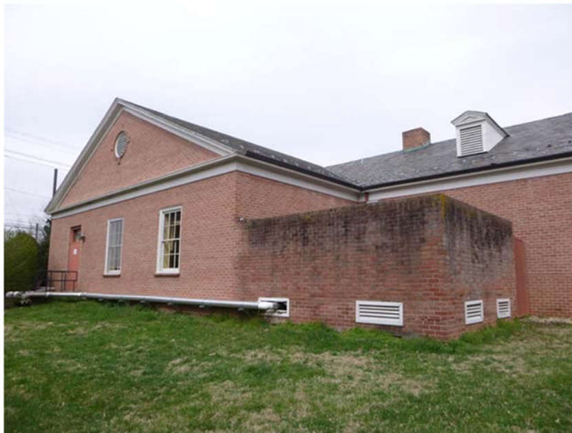
Photo 11: Partial view of the southeast elevation. Note the staining on the screen wall. The mortar throughout is in generally deteriorated condition.
