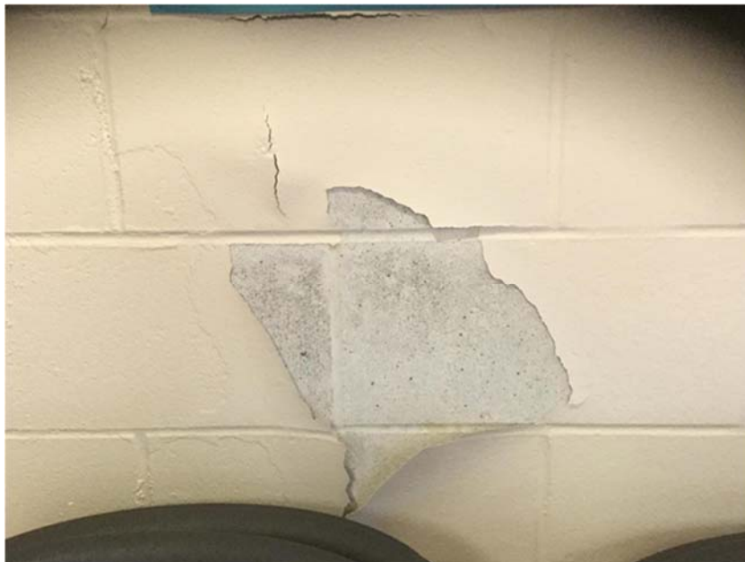
Photo 2: Typical peeling paint and efflorescence observed on the north and south CMU walls in the lower level meeting room.
