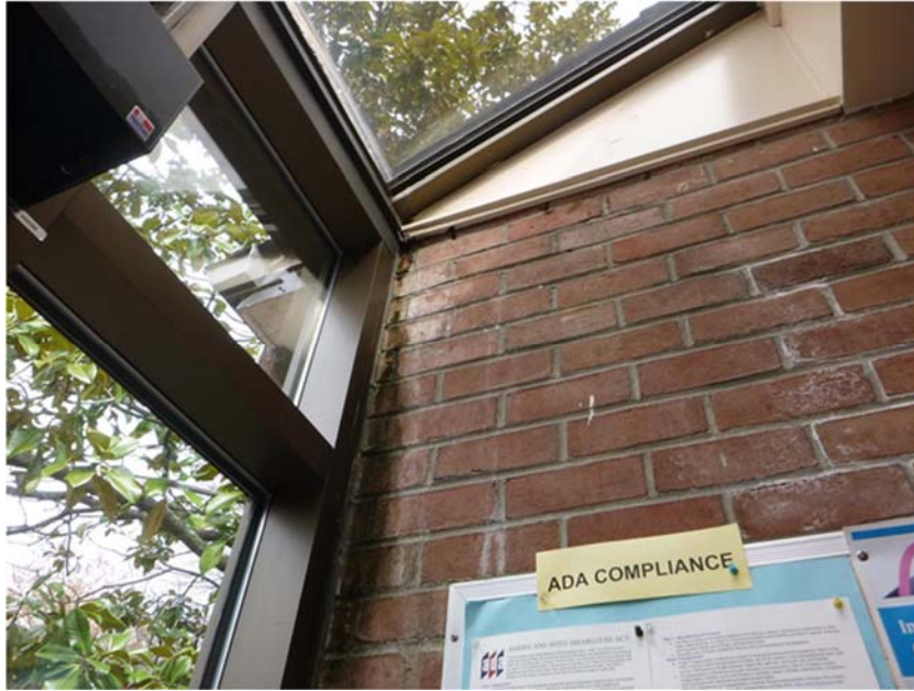
Photo 15: View of staining on interior brick, indicative of moisture intrusion from the curtainwall.
