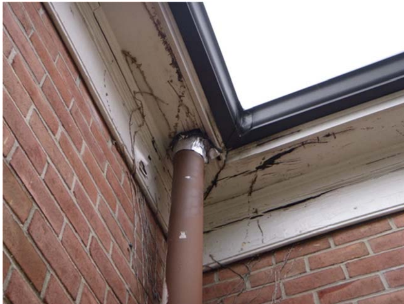
Photo 10: Downspout shown in Photo 8. Peeling paint and isolated rot noted throughout the fascia assembly. Note the repairs at the downspout.
