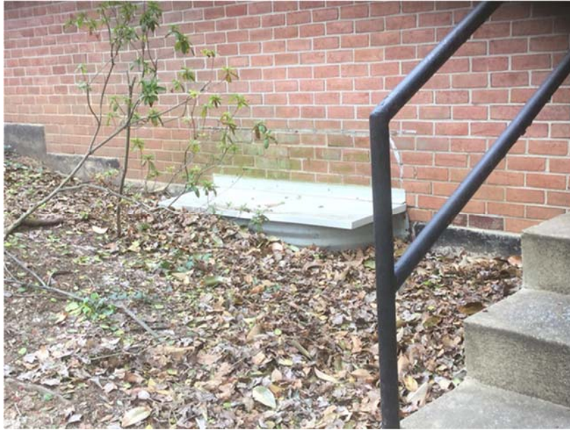
Photo 17: Parge coating with dampproofing was noted throughout the building exterior.
