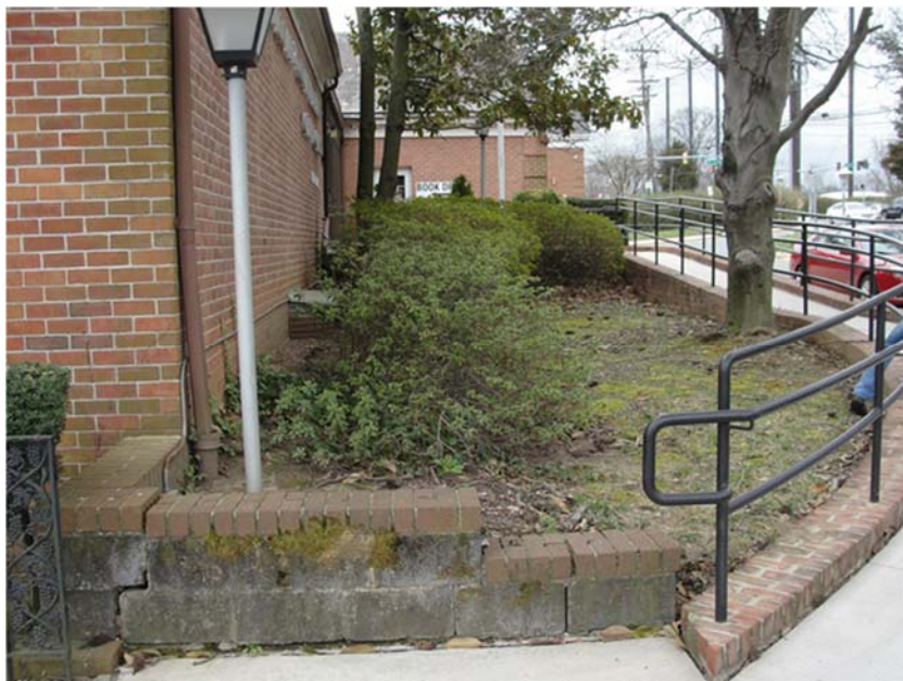
Photo 18: Note the garden wall and ramp prevent drainage of the landscaping area. See Photo 2 for correlating defects on the meeting room walls.
