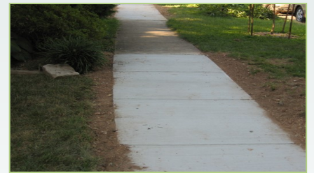
Completed sidewalk repair
