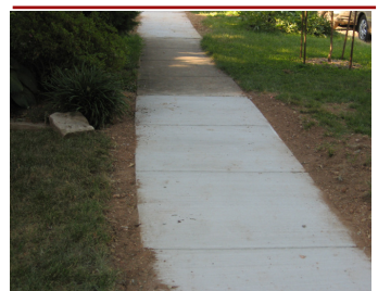
Completed sidewalk repair
