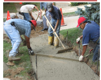
Concrete is smoothed and finished
