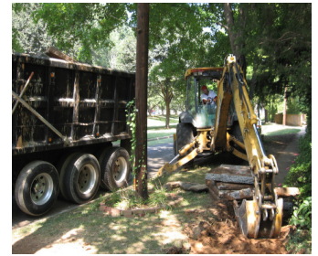
Defective concrete is removed
