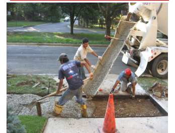
New concrete is poured into forms
