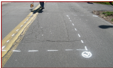
Typical paint markings
