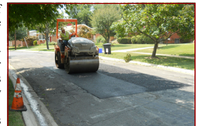
New asphalt is placed and compacted
