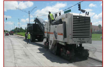
Milling machine excavating
