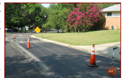
New patch is flush with existing pavement
