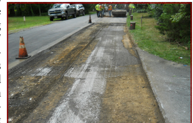
Pavement will be replaced in 2 phases
