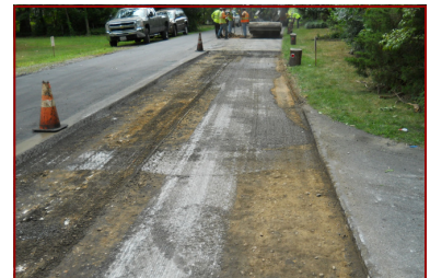
Pavement will be replaced in 2 phases
