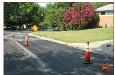
New patch is flush with existing pavement
