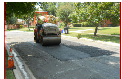
New asphalt is placed and compacted
