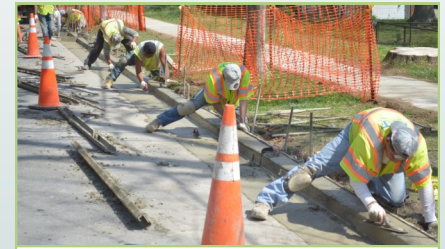
Concrete is smoothed and finished
