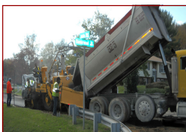
Typical asphalt paving operation.
