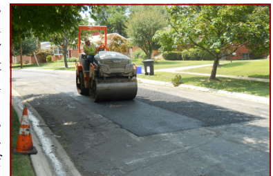
New asphalt is placed and compacted
