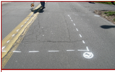
Typical paint markings
