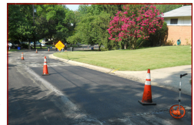
New patch is flush with existing pavement
