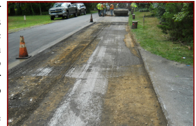
Pavement will be replaced in 2 phases
