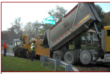
Typical asphalt paving operation.
