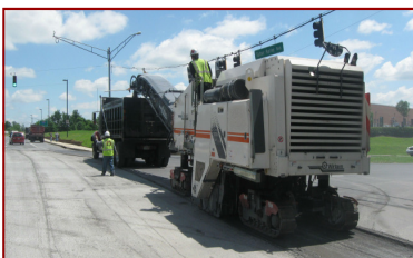
Typical milling (pavement excavating) operation.
