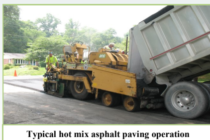
Typical hot mix asphalt paving operation
