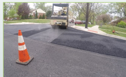
New asphalt is placed and compacted
