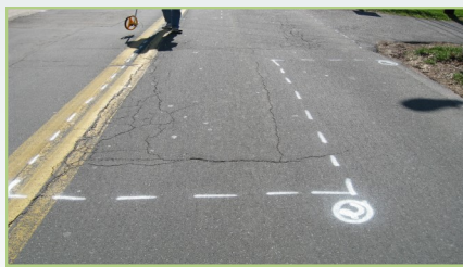
Typical survey paint markings
