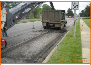
Typical milling operation
