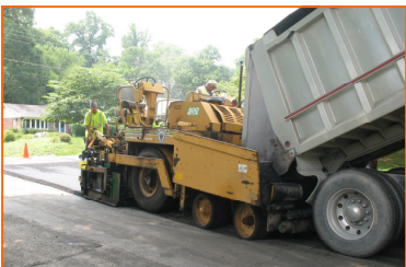
Typical asphalt paving operation
