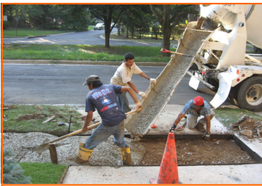
Pouring new concrete into forms
