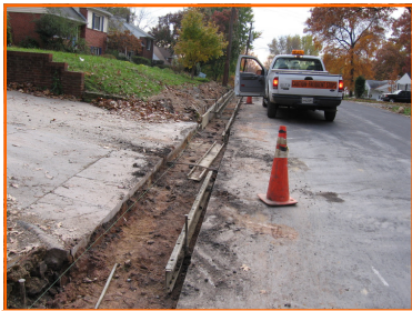
Curb forms ready for concrete
