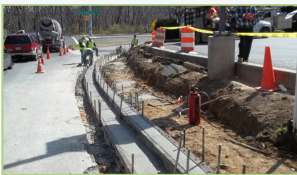
New concrete is poured into forms
