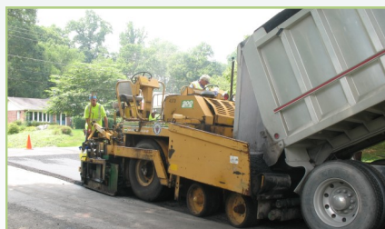
Typical asphalt paving operation
