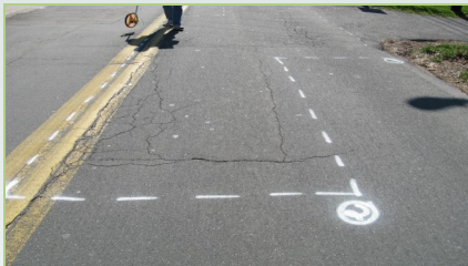
Typical survey paint markings
