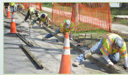
Concrete is smoothed and finished
