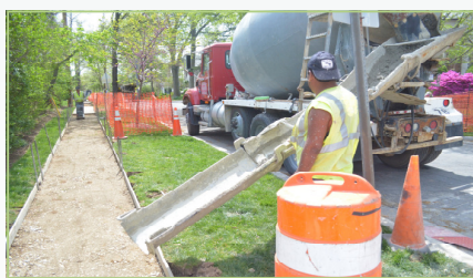
New concrete is poured into forms
