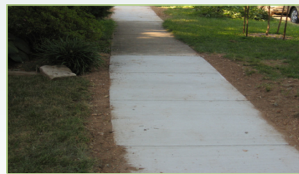
Completed sidewalk repair
