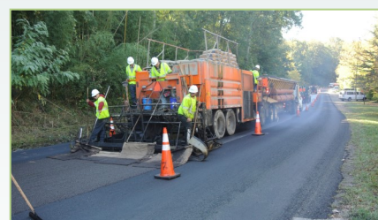
Typical micro-surfacing operation
