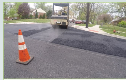
New asphalt is placed and compacted
