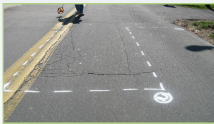
Typical survey paint markings
