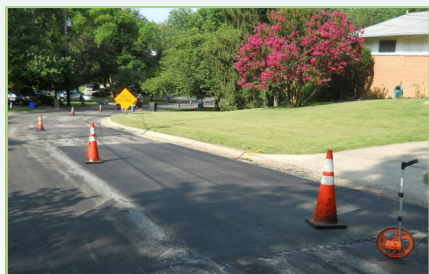
New patch is flush with existing pavement
