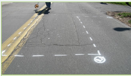
Typical survey paint markings
