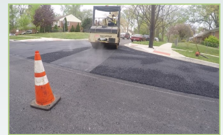
New asphalt is placed and compacted
