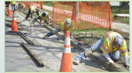
Concrete is smoothed and finished
