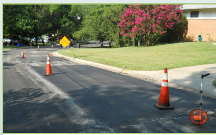
Example of completed patching
