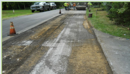
Patching will precede resurfacing by several weeks
