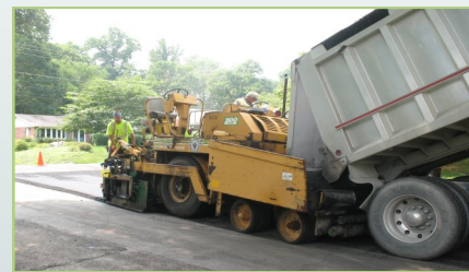
Typical hot mix asphalt paving operation
