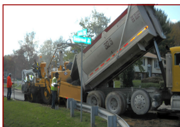
Typical asphalt paving operation.
