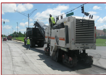
Typical milling operation.
