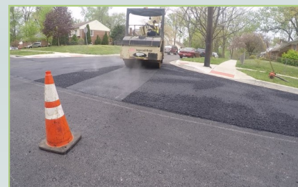
New asphalt is placed and compacted
