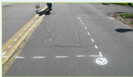
Typical survey paint markings
