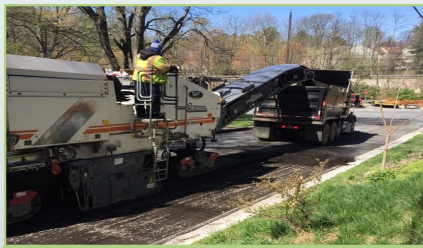
Milling machine patch excavating
