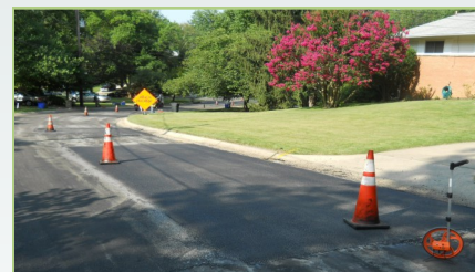
New patch is flush with existing pavement
