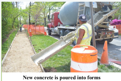
New concrete is poured into forms
