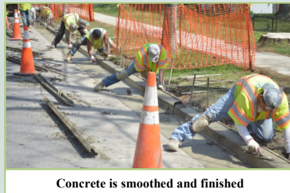
Concrete is smoothed and finished
