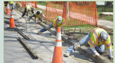
Concrete is smoothed and finished
