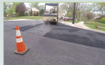
New asphalt is placed and compacted
