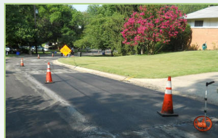
New patch is flush with existing pavement
