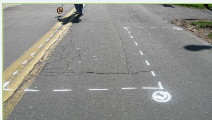
Typical survey paint markings
