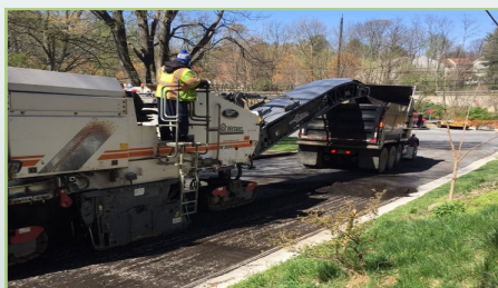
Milling machine patch excavating
