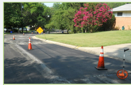
New patch is flush with existing pavement
