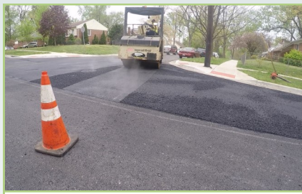
New asphalt is placed and compacted
