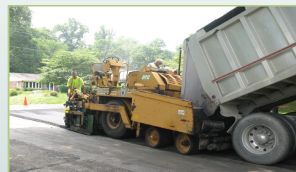
Typical hot mix asphalt paving operation
