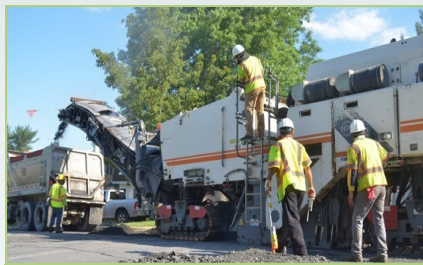
Typical milling operation
