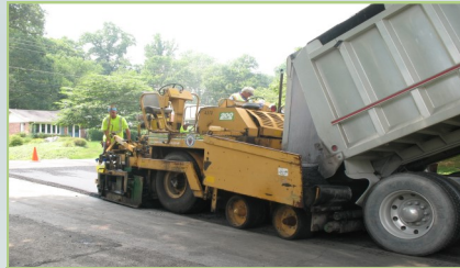
Typical hot mix asphalt paving operation
