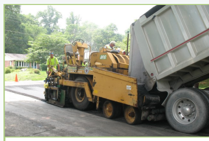
Typical asphalt paving operation
