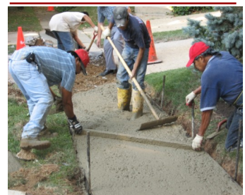
Concrete is smoothed and finished
