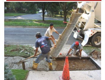
New concrete is poured into forms
