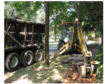
Defective concrete is removed
