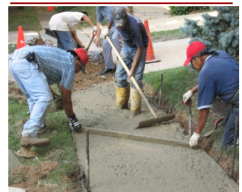
Concrete is smoothed and finished
