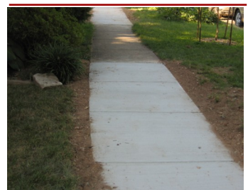
Completed sidewalk repair
