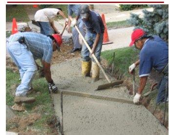
Concrete is smoothed and finished
