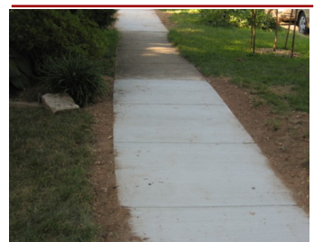
Completed sidewalk repair
