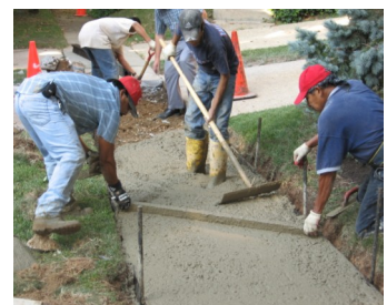
Concrete is smoothed and finished
