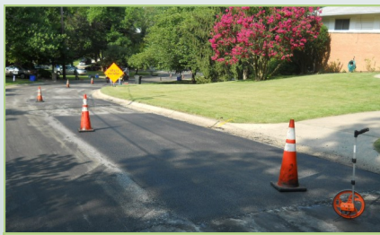
Example of completed patching
