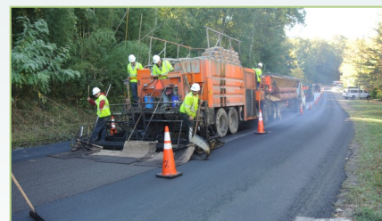
Typical micro-surfacing operation
