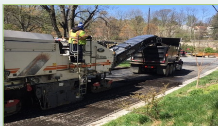
Milling machine patch excavating
