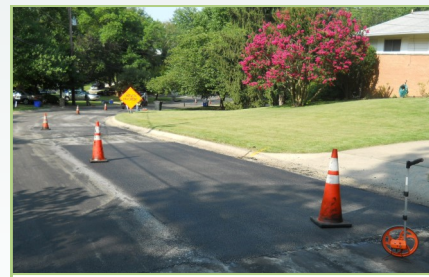
New patch is flush with existing pavement
