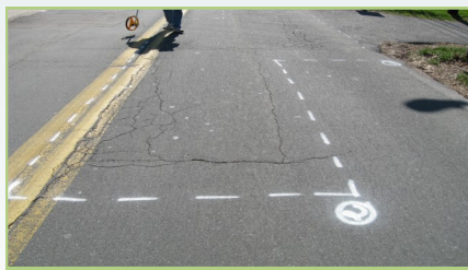
Typical survey paint markings
