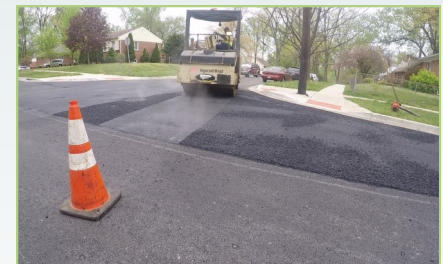
New asphalt is compacted with steel wheeled roller
