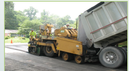
Typical hot mix asphalt paving operation
