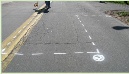
Typical survey paint markings
