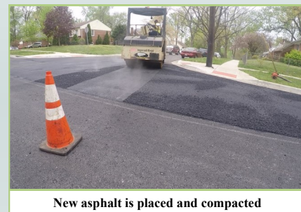
New asphalt is placed and compacted
