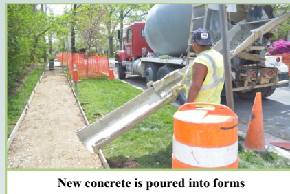
New concrete is poured into forms
