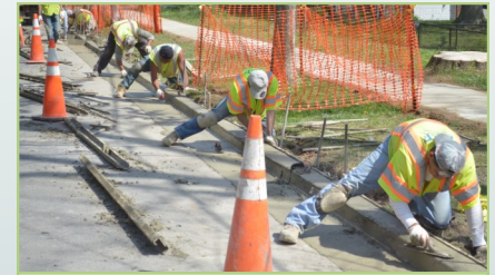
Concrete is smoothed and finished
