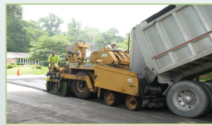
Typical hot mix asphalt paving operation
