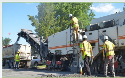
Typical milling operation
