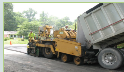
Typical hot mix asphalt paving operation
