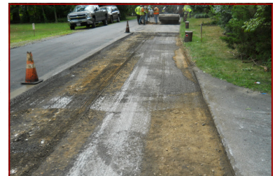
Pavement will be replaced in 2 phases
