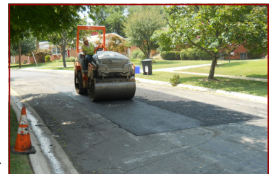
New asphalt is placed and compacted
