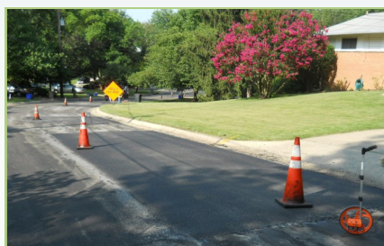
New patch is flush with existing pavement
