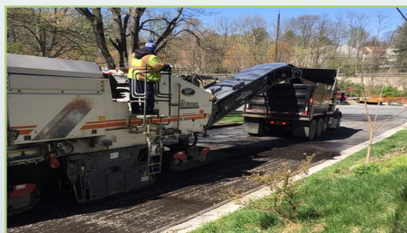
Milling machine patch excavating
