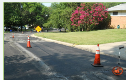
New patch is flush with existing pavement
