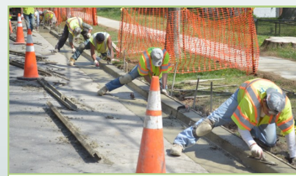
Concrete is smoothed and finished
