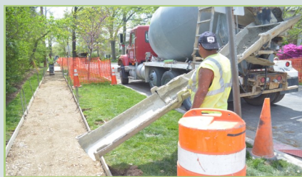
New concrete is poured into forms
