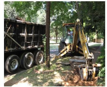
Defective concrete is removed
