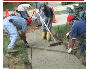
Concrete is smoothed and finished
