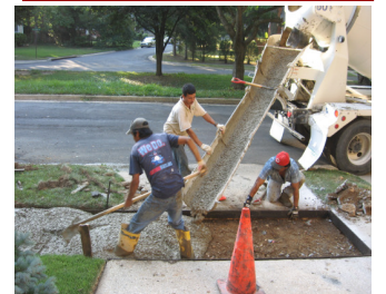
New concrete is poured into forms
